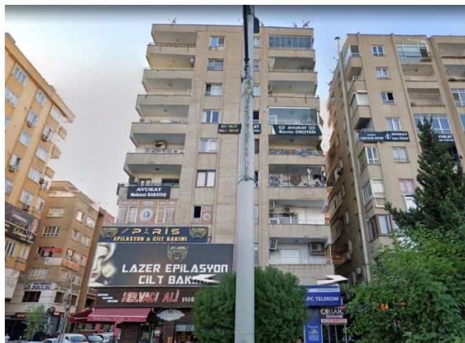
◆ Before image of the destroyed building (Google street view)
